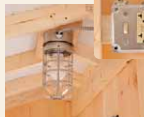
Electric Package Switch / Outlet / Lights Extension Cord Hookup
