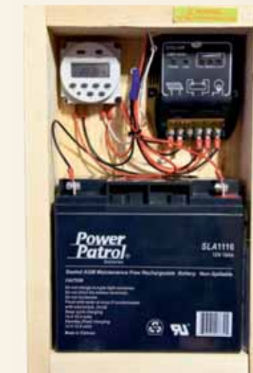
Inside view of control box
