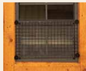
Wire over window
