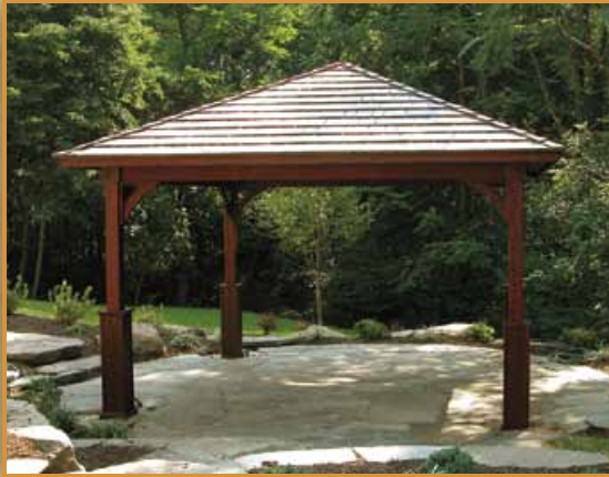
Large Roof Overhang
