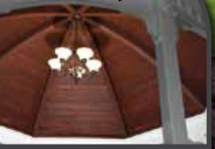
Underside of Bell Roof
