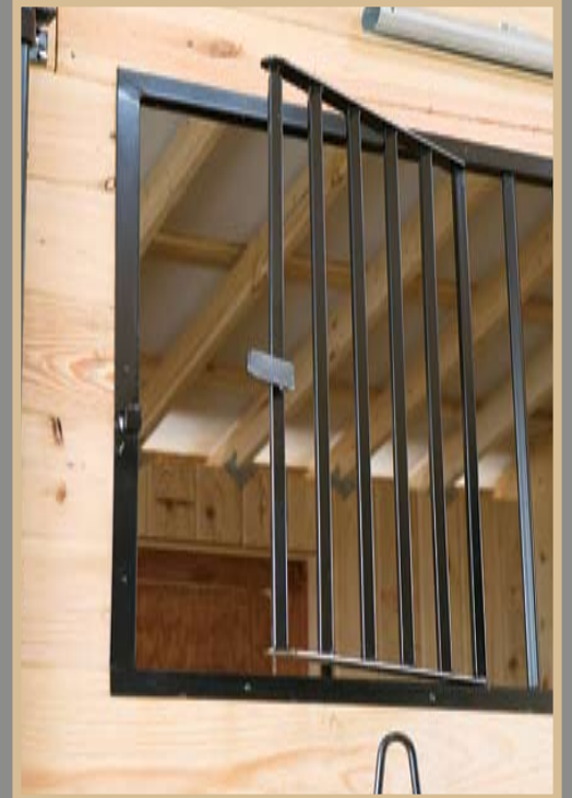
STALL FRONT GRILL FOR FEED ENTRY
