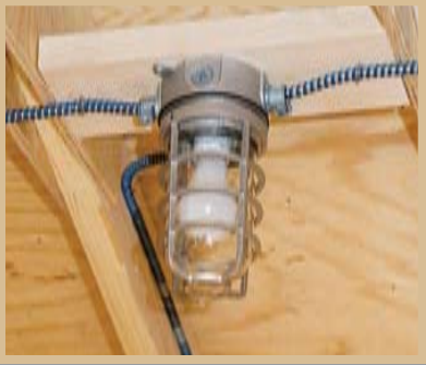
VAPOR PROOF LIGHTS WITH DIE CAST GUARD
