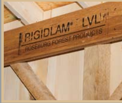
GLUE LAM LVL HEADER FOR INCREASED SNOW LOADS & HURRICANE REGIONS
