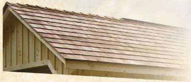
Cedar Shake Roof
