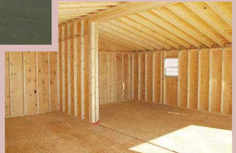
Interior View of 24' x 28' Double Wide (below)
