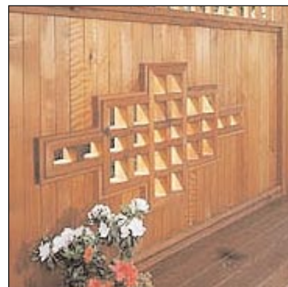
Clockwise from top: a simple inset board-and-board fence encloses a patio; 2x4 wall treatment allows filtration of light and air through to a spa and deck; craftsman style gate with an open trellis creates an inviting entrance.
